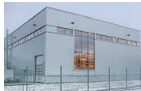
AK-Tehdas Oy's plant extension in Tampere.
